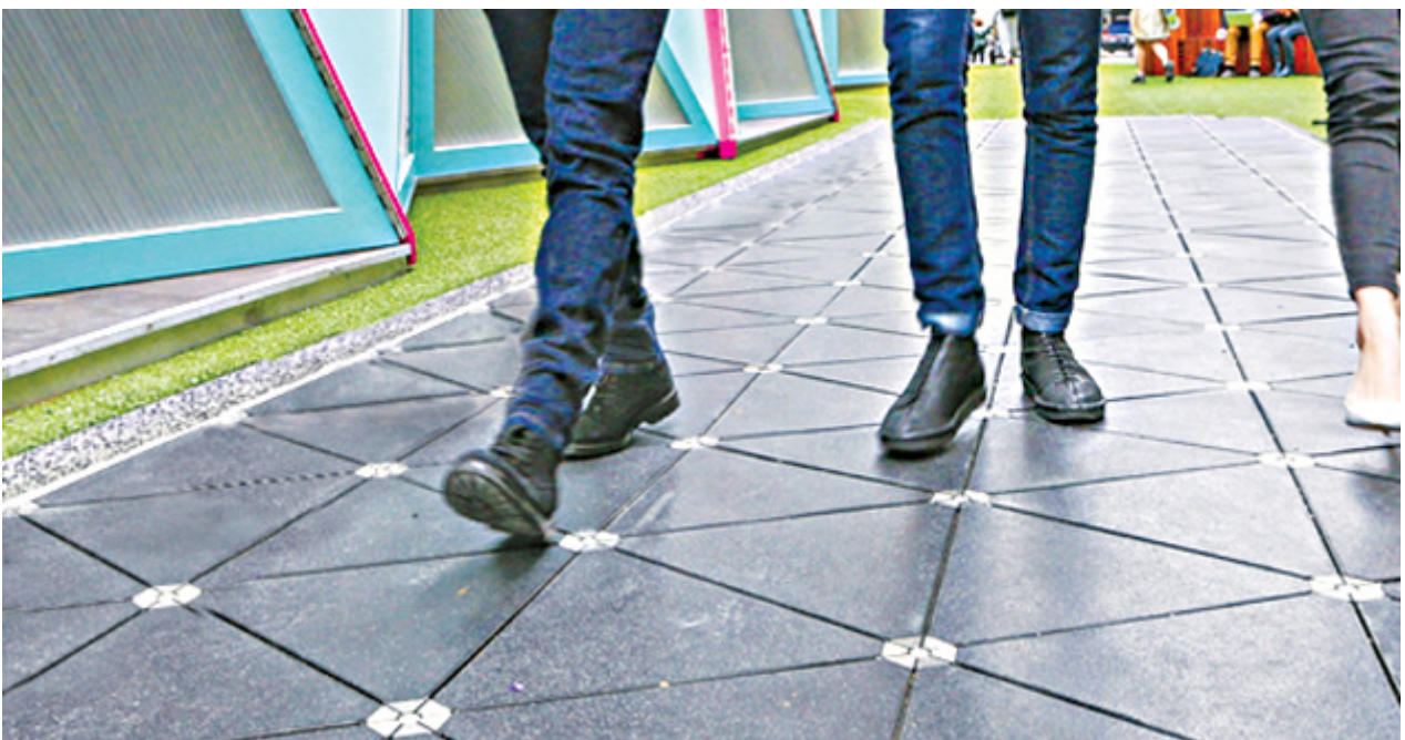
Pavegen's tech captures energy from pedestrian footsteps to power street lighting. (Supplied)
