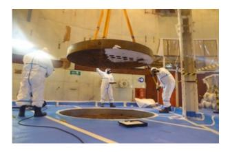
DMTR became Scotland's first operating reactor when it achieved criticality in 1958. It was used for irradiation tests on materials until its shutdown in 1969. In 2018 a contract was awarded to Cavendish Nuclear Limited to dismantle and demolish the reactor. The fuel, heavy-water coolant and some redundant plant have been removed, leaving the reactor vessel, supports and containment shell ready for final demolition.
