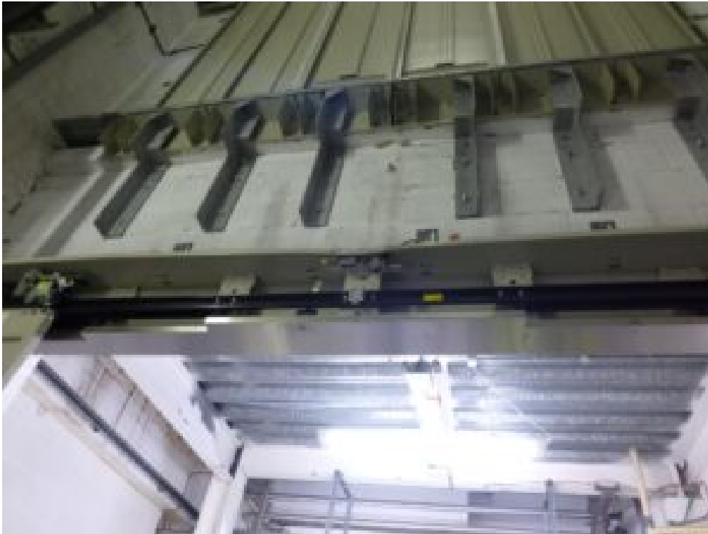
The lift shaft wall
