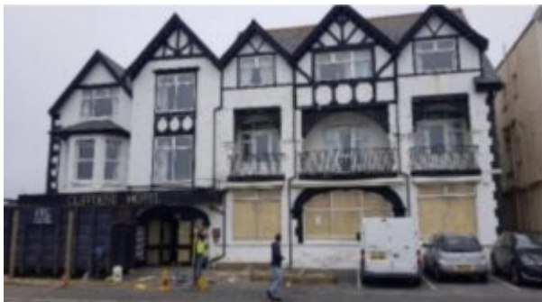
The former Cliffdene Hotel in Newquay
