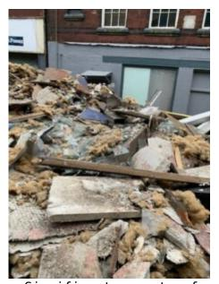
• Significant amounts of asbestos-containing debris to the front and rear of the building and along the public highwayconstructio
