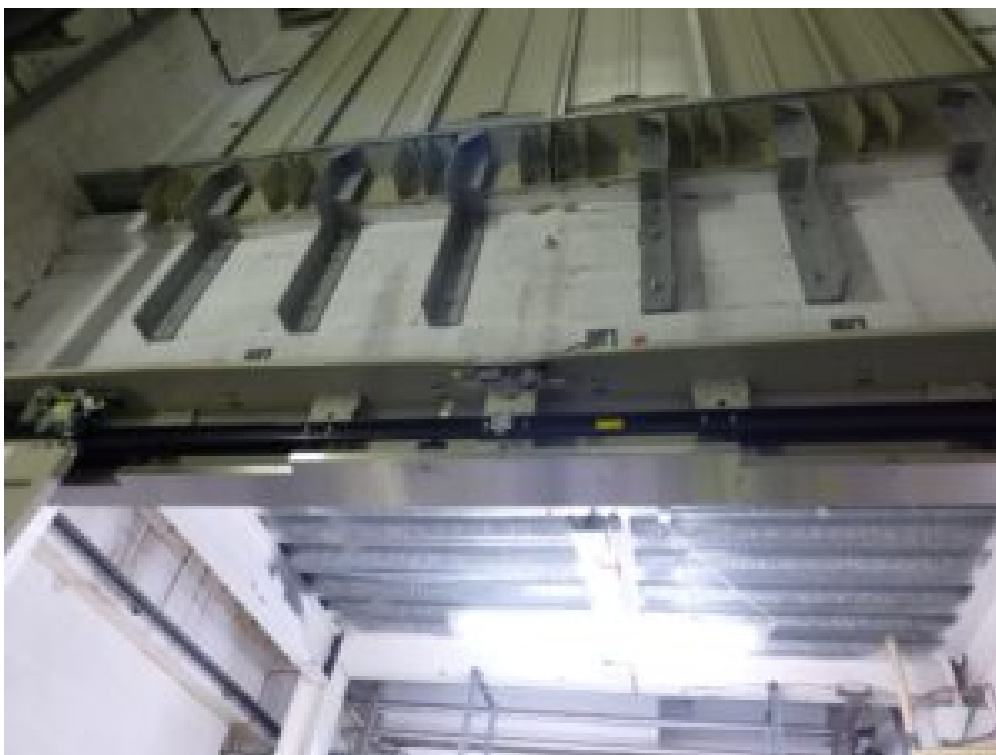
The lift shaft wall
