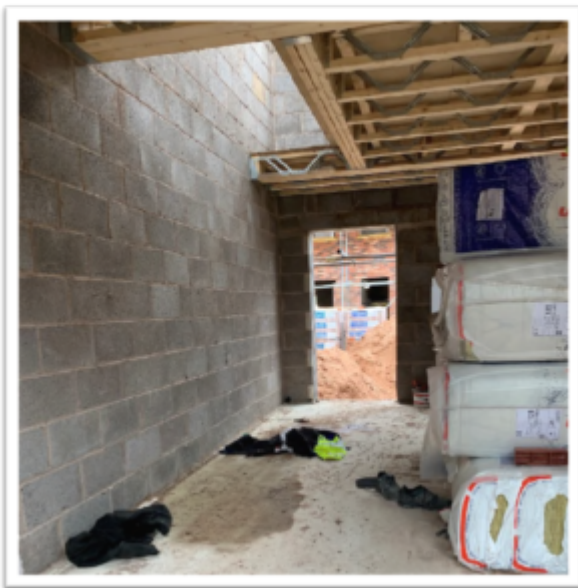
The open stairwell
