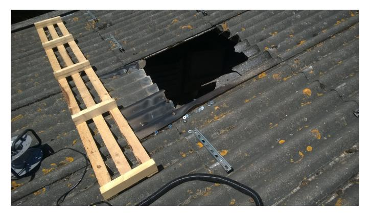
An investigation by the Health and Safety Executive (HSE) found that, although the company knew the risks from fragile surfaces and unprotected edges, they failed to plan or supervise the work to ensure that access to hazardous areas was prevented. As such the workers were at risk from falls throughout the job.
