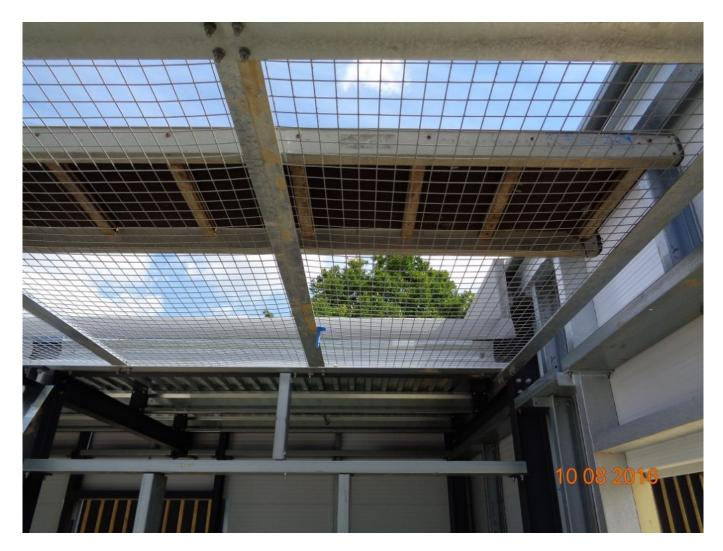
The Health and Safety Executive (HSE) investigation found that in failing to prevent access to the fragile roof area, the roofing contractor, Metcalfe Roofing & Building Services Limited, had failed to plan and carry out the work at height in a safe manner. The investigation also found the principal contractor, P.D.R. Construction Limited, had failed to plan, manage or monitor an aspect of the construction phase without risk to safety.
