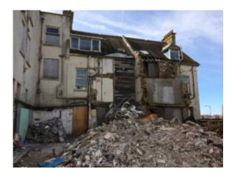
During a proactive inspection, the Health and Safety Executive (HSE) identified that the former hotel was being refurbished and partially demolished whilst ACMs remained in-situ. Some of these ACMs were licensable products (e.g. asbestos insulating board which contains amosite). Due to the extent of the spread of asbestos dust and debris throughout the building and the lack of adequate control measures, workers and visitors to the properties were at risk of exposure to asbestos fibres.
