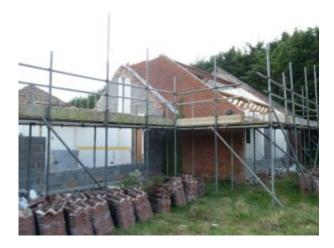
Portsmouth Crown Court heard how David Shayler, an employee of Ryde Demolition Limited, was removing roof timbers by hand with a colleague, when a gable wall partially collapsed causing him to fall backwards striking his head against a stack of roof tiles.
