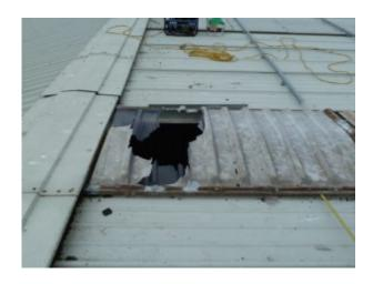
An investigation by the Health and Safety Executive (HSE) found that the fall from height was possibly due to the unsafe working environment and unsafe methods of working being undertaken. It was established the main cause of the incident was insufficient identification of risk in the work being done.
