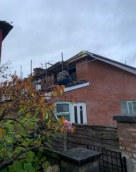
Mr Rehman working on lower roof himself in November 2021
