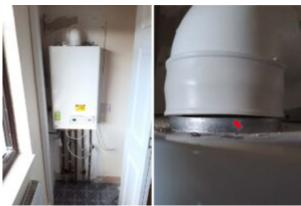
The new LPG boiler was fitted with a securing clamp missing from the chimney/flue with a gap clearly visible
