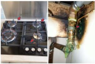
The gas hob which was found to be 'immediately dangerous' with a yellow flame due to improper combustion. Bubbles can also be seen emanating from the solder joint underneath the hob.
