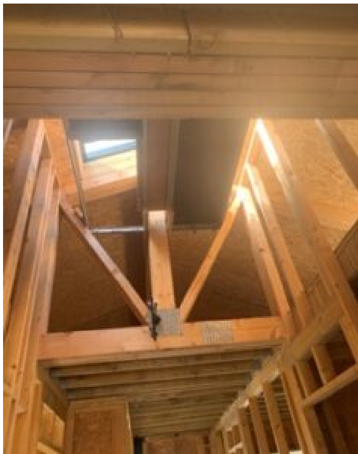
View of the roof inside the property
