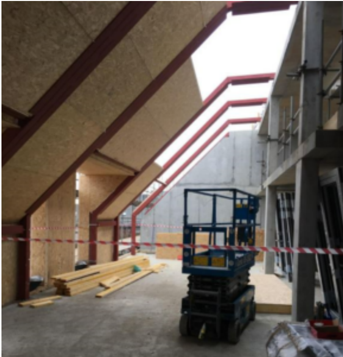
The construction site at Eskdale Terrace, Jesmond, Newcastle
