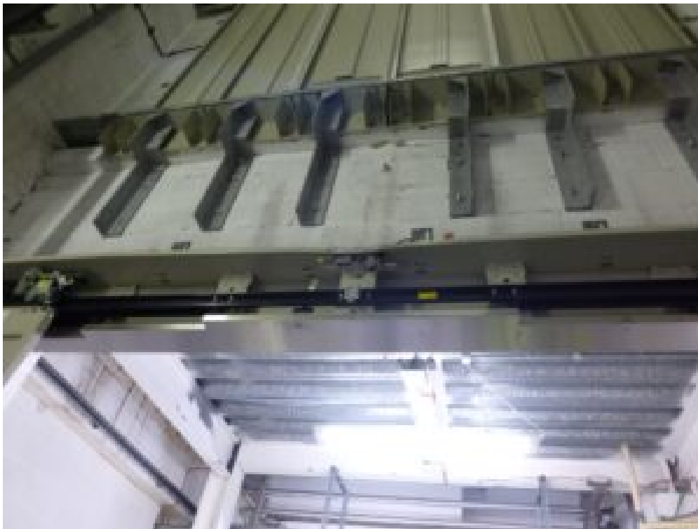
The lift shaft wall
