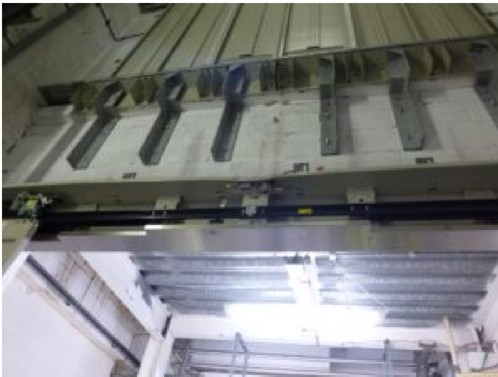
The lift shaft wall
