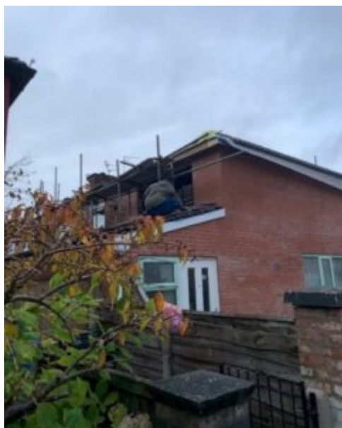
Mr Rehman working on lower roof himself in November 2021
