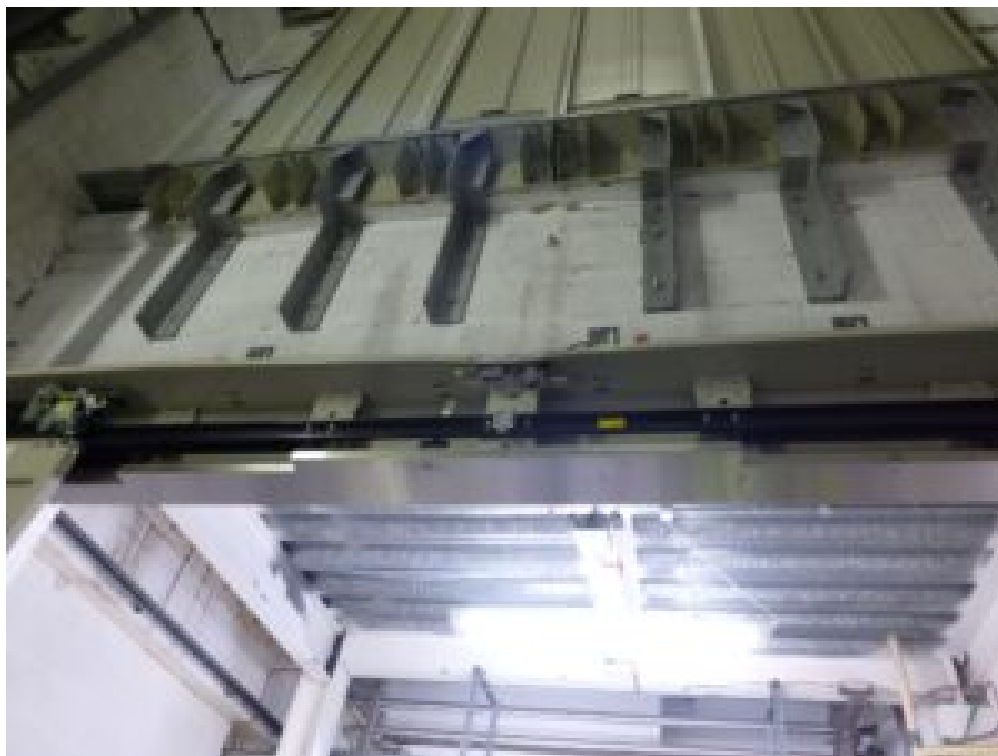
The lift shaft wall
