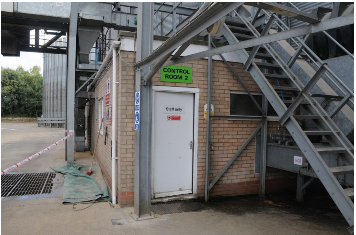
Image showing no barrier segregating personnel from vehicles
