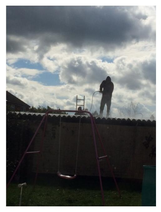
An investigation by the Health and Safety Executive (HSE) found that work should have been planned to include the use of basic precautions as detailed in published and widely recognised guidance for working with asbestos cement. Low energy cleaning methods and proper protective measures would have prevented the release of asbestos fibres thus eliminating much of the risk.
