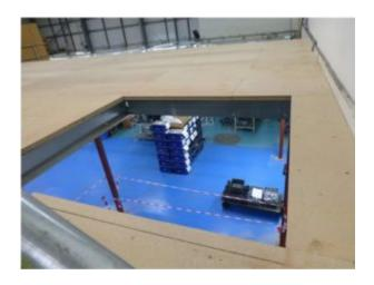
An investigation by the Health and Safety Executive (HSE) revealed that the contractor failed to adequately plan, manage and monitor the construction work, so as to ensure that appropriate methods to prevent or mitigate a fall during the construction work, were in use.
