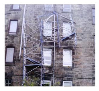
Glasgow Sheriff Court heard that, on 2 September 2016, work was undertaken at a four-storey property in Alexandra Parade in Glasgow to erect a tower scaffold to repair a roof. An employee was fitting toeboards to a cantilever section attached to the tower scaffold and the tower partially collapsed causing him to fall eight metres to the ground below.
