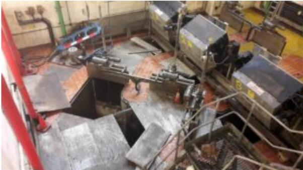
Edinburgh Sheriff Court heard how, on 9 June 2017, an employee of Scottish Water entered into the screen well area at Prestonpans Pumping Station and fell through the insecure floor panels into a sewage filled storm channel some 3.1 metres below.
