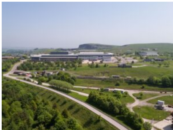
HSE's Buxton Science and Research Facility from the Air
