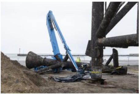
The skirt pile gave way and struck a mobile elevating work platform
