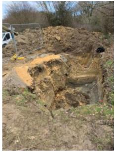
The three men were working in this excavation when it collapsed
