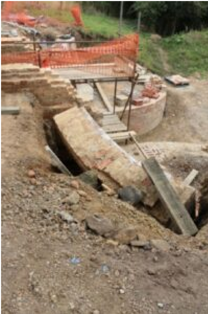
A section of the wall collapsed while Mr Konitzer was inside the excavation
