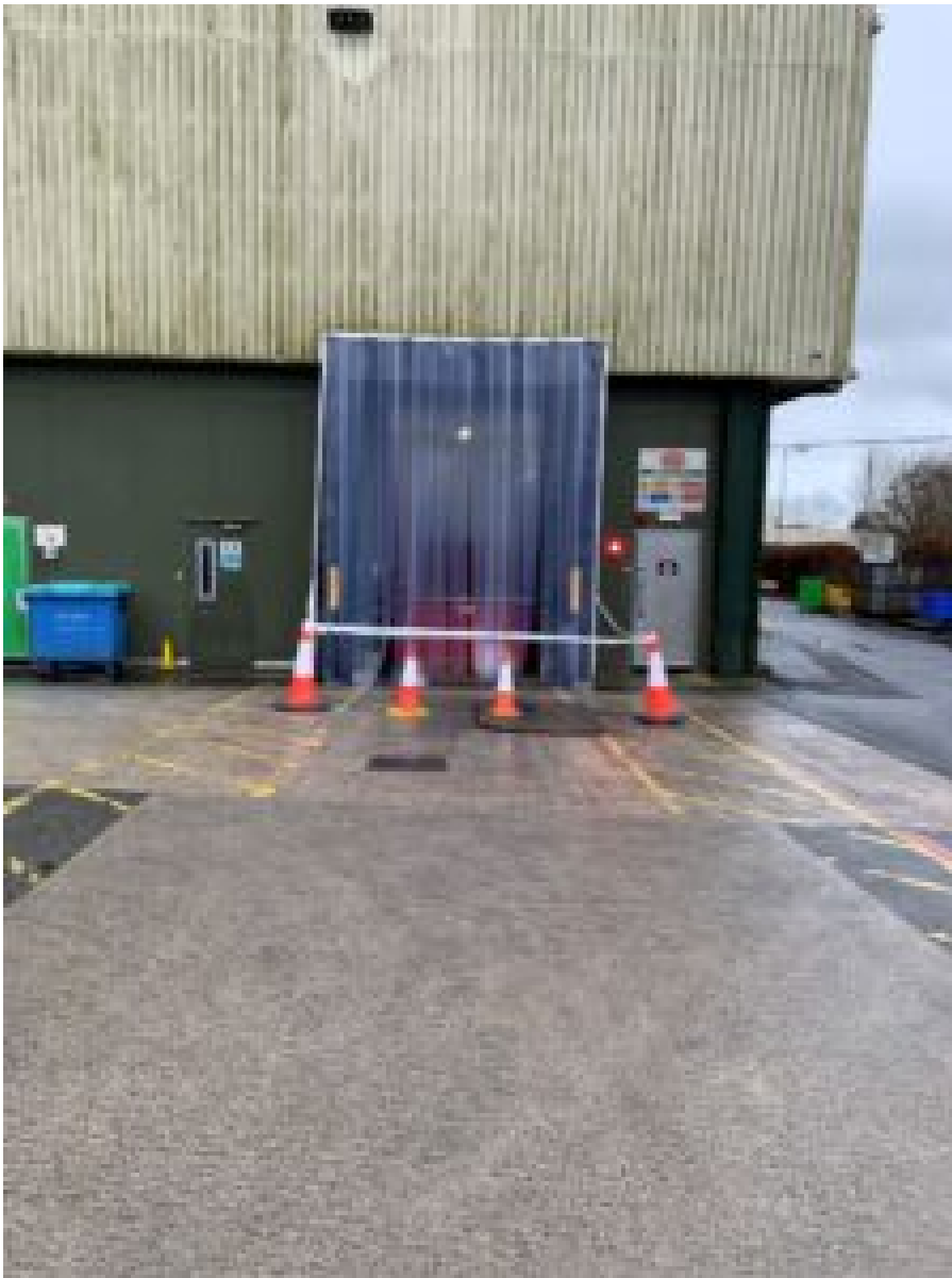
The intake bay where the incident occurred
