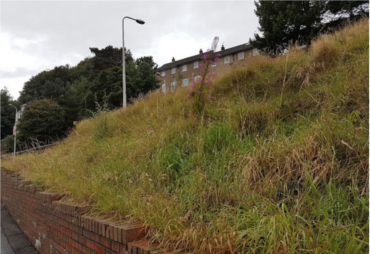
West end of Scott Street
