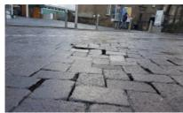
I have expressed concern that, <u>less than a year</u> after the resurfacing and relaying of the block paving surface at Nethergate outside Dundee Contemporary Arts, the road surface is already appearing to sink in places and is uneven – see right:
