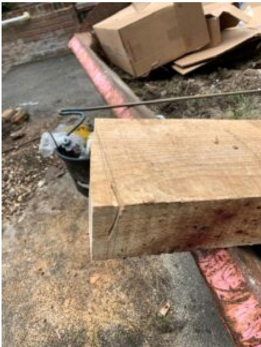
The sleeper had been placed in a skip and was not secured whilst being cut.
