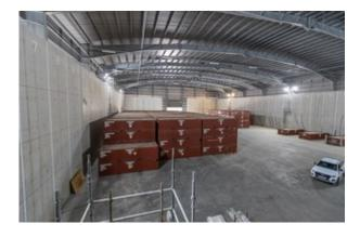
As part of the waste disposal process, the spaces between the containers in the low level waste vault are being filled with grout.
