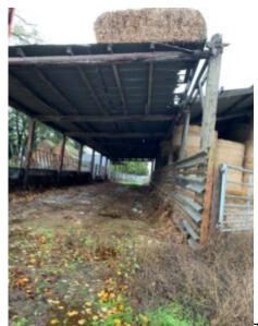
The HSE investigation found one of the barns used as an employee through route was deemed unsafe to enter due to its poor structural state. Seymour Stevens Ltd were aware of this but had decided not to repair the shed due to costs. A number of electrical faults were also identified.
