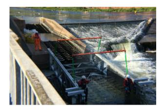
The 7.3m extension to the Trews Weir fish pass is bolted into place
