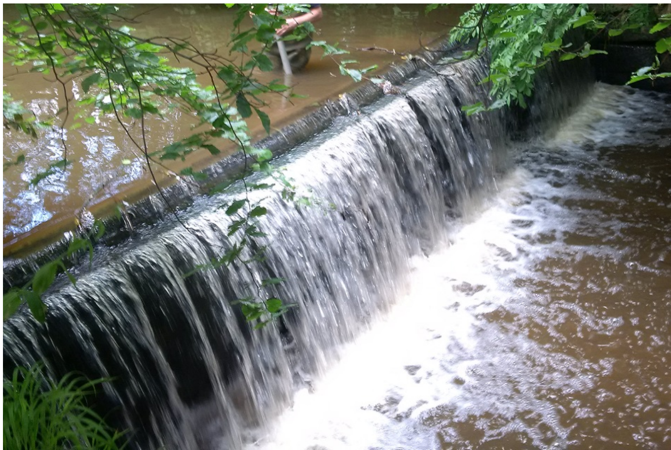
Upstream weir before it was altered to make it easier for fish migration
