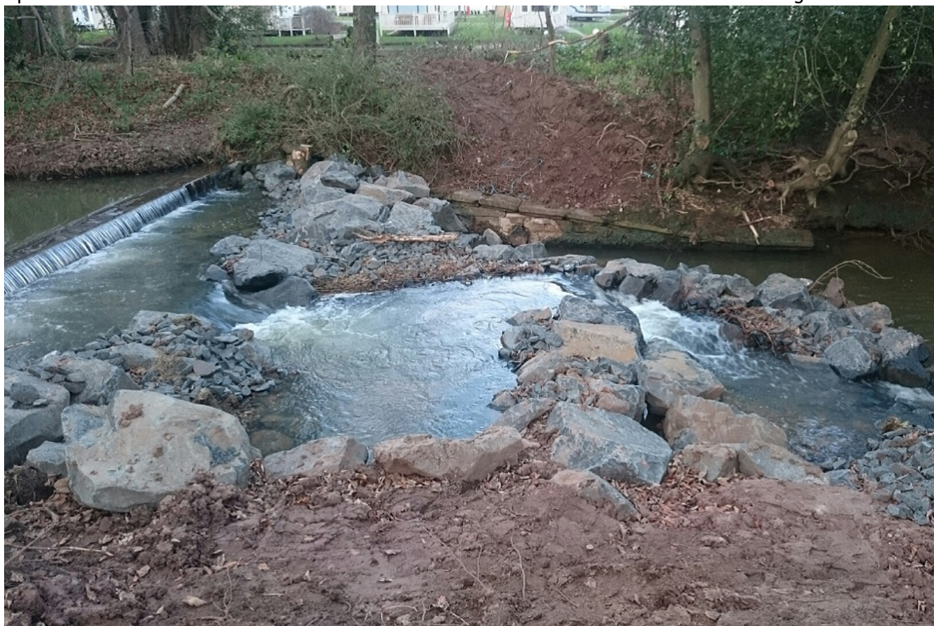
The new upstream fish pass after alterations were made to the weir to make it
