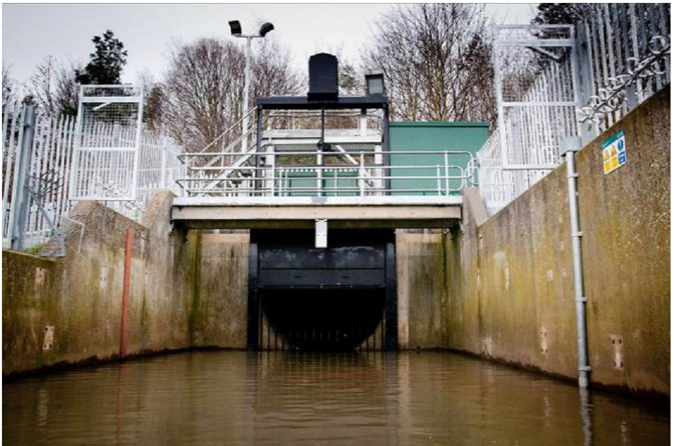
The lifting screen at Primrose Hill
