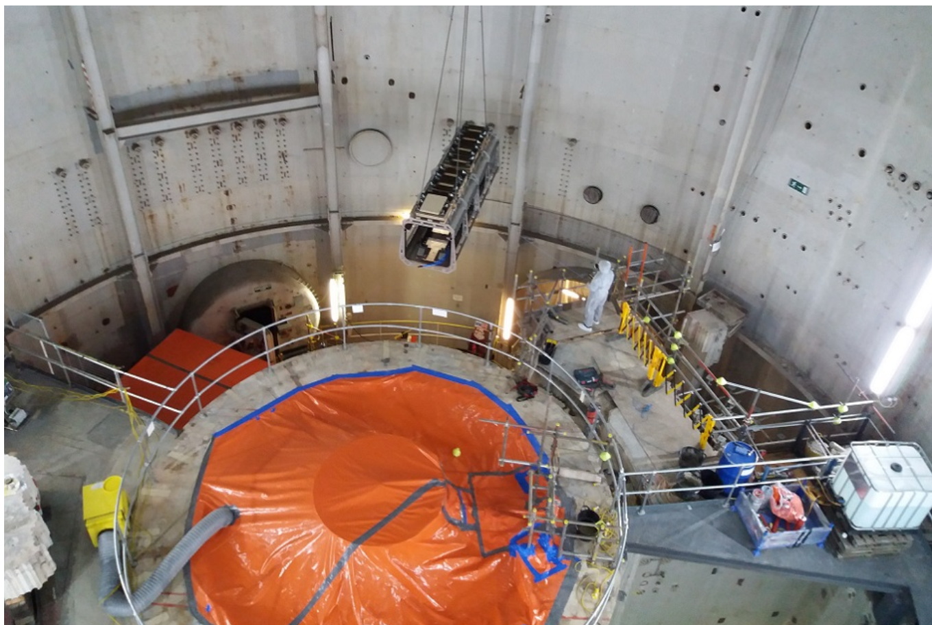
LaserSnake and its housing are lifted into place at the Dragon reactor
