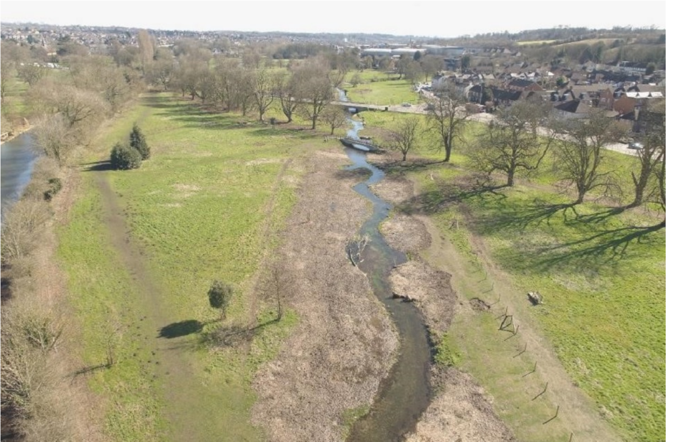
An aerial photo showing the restored river after the project works.
