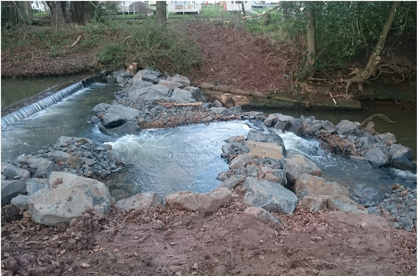
The new upstream fish pass after alterations were made to the weir to make it into a rock pass
