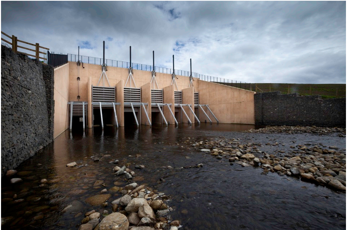
The large dam at Mitford
