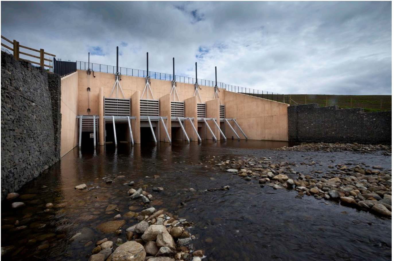
The large dam at Mitford
