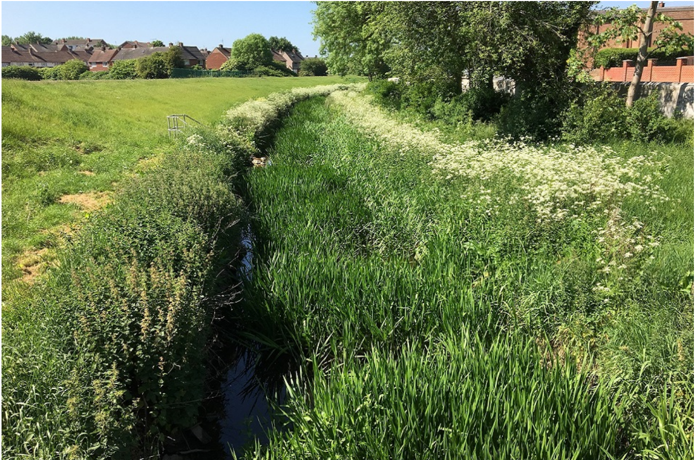
Lustrum Beck: Raised embankment (L) and new flood wall (R)
