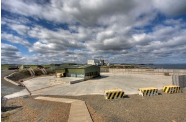
The Dounreay shaft
