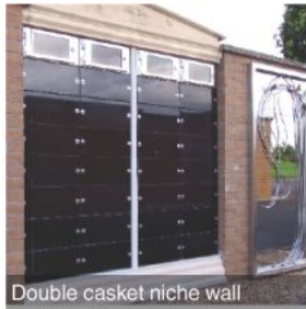
Double casket niche wall
