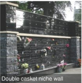
Double casket niche wall
