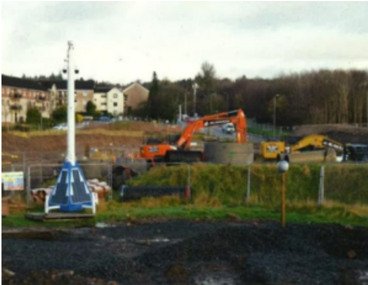
The construction site adjacent to Glenkirk Drive
