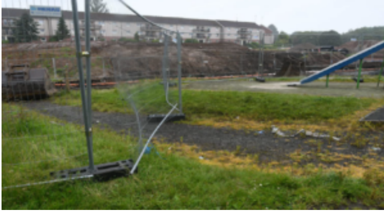
The construction site adjacent to Glenkirk Drive
