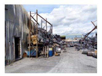
An investigation by the Health and Safety Executive (HSE) found that the process involved placing a bulk container of heptane onto racking at a height of about 1.5m. A table was then positioned beneath the bulk container onto which a small electrical weighing scale was positioned. Metal cans were placed onto the scale and an employee filled the cans by weight by manually operating a tap on the bulk container in the warehouse building.
