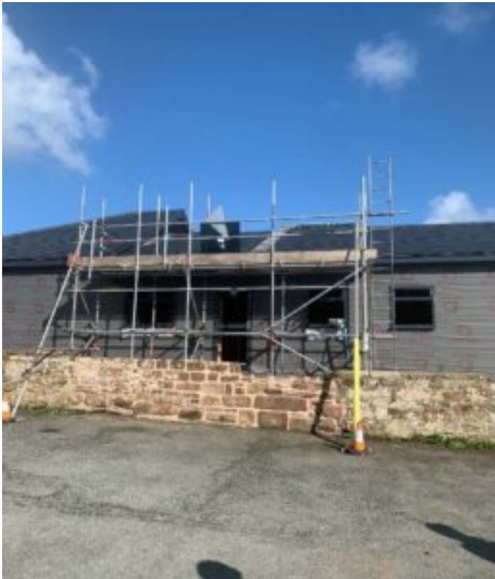
The site on Village Lane, Frodsham, Cheshire
