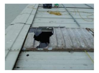
An investigation by the Health and Safety Executive (HSE) found that the fall from height was possibly due to the unsafe working environment and unsafe methods of working being undertaken. It was established the main cause of the incident was insufficient identification of risk in the work being done.
